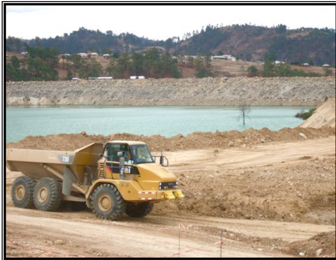
Figure 1: Tailings pond at the Marlin Mine.
